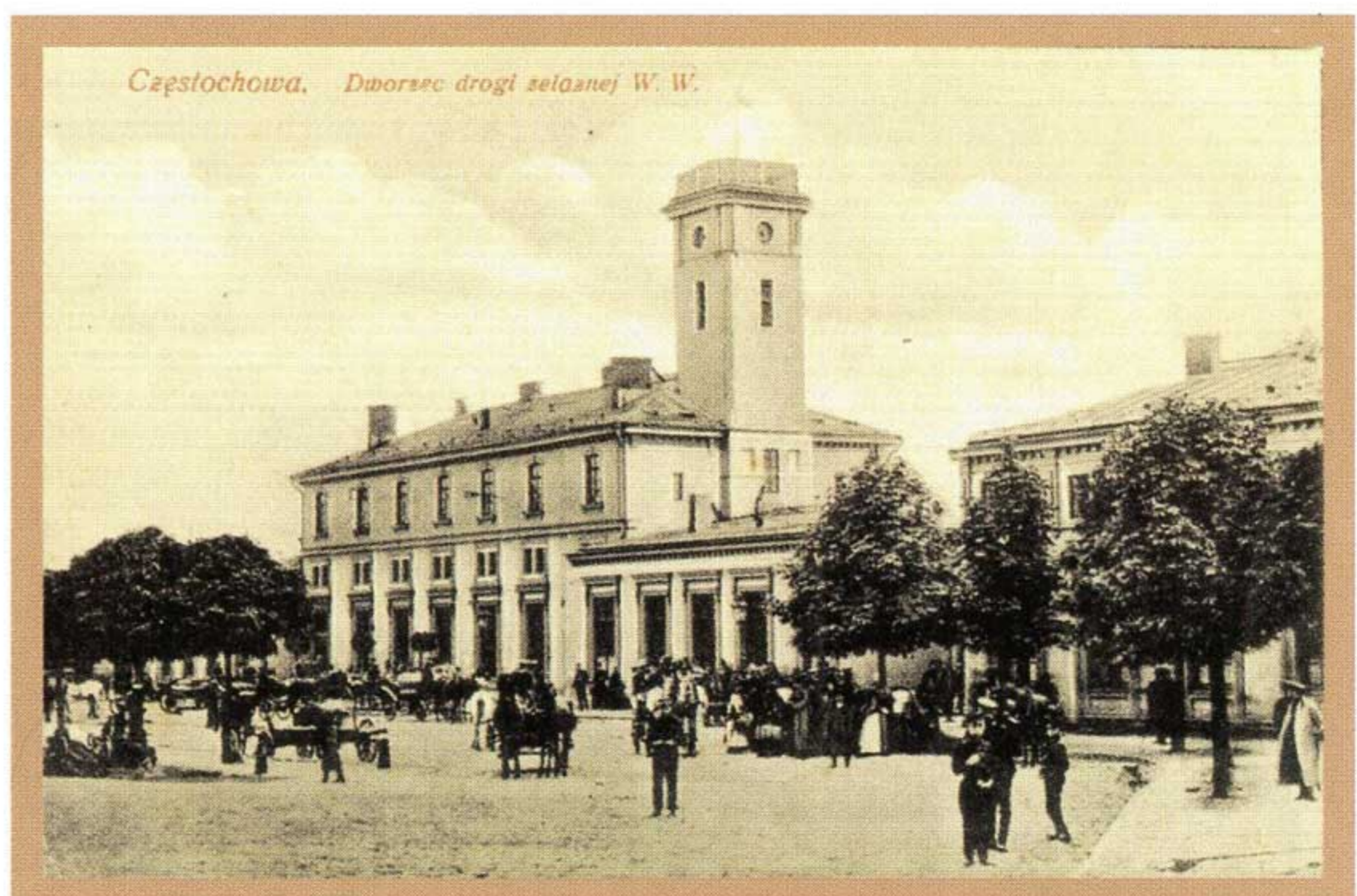
Warsaw-Vienna railroad terminal, c. 1917
